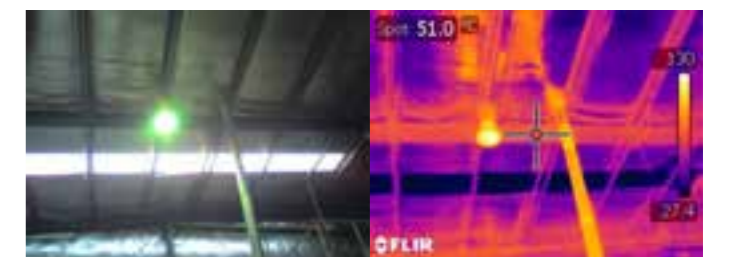
Temperatures of up to 51°C was recorded for the roof space, triggering false fire alarms.
